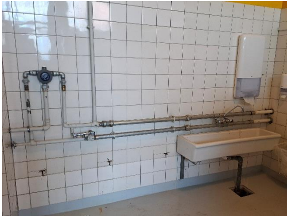
Vandinstallation i baderum
