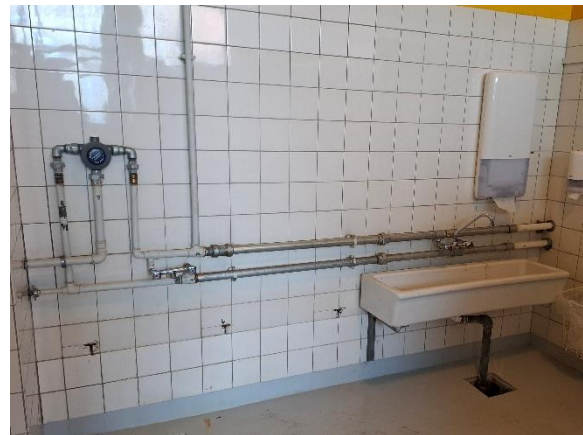
Vandinstallation i baderum
