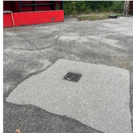
Afvandingsbrønd (ristbrønd)
