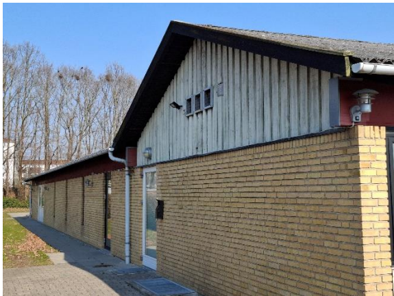
Murede facader mod vest
