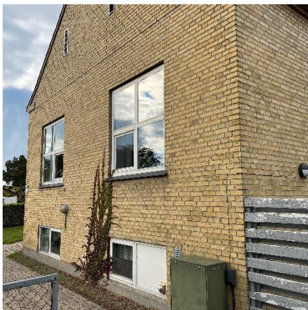
Murstensfacade i gavl
