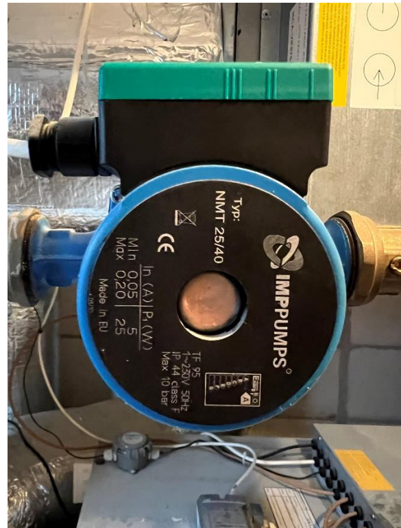
Gammel NMT pumpe, 25 W.
