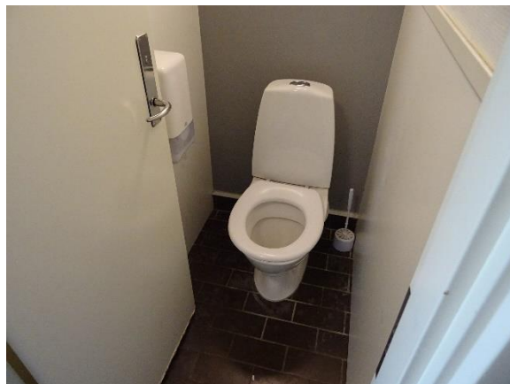
Nyere to skylds toilet
