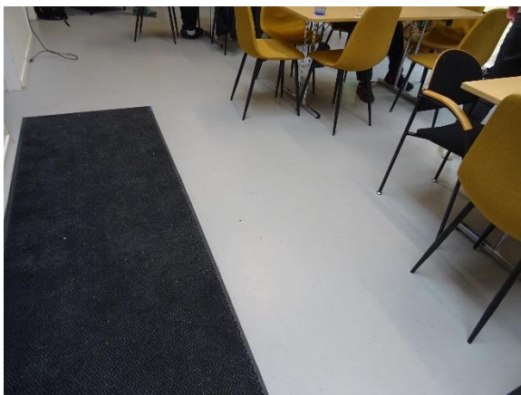
Gulve i epoxy
