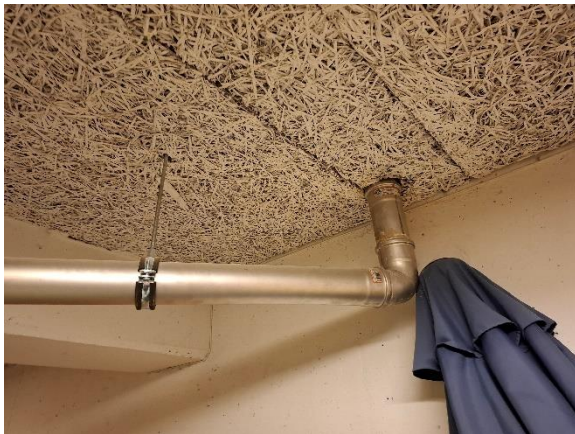
Ny installation i rustfast stål
