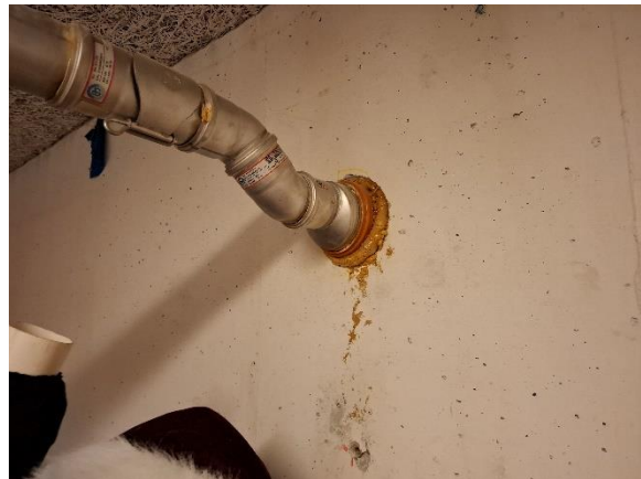
Ny installation i rustfast stål
