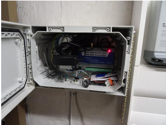
GSM modul for pumpealarm
