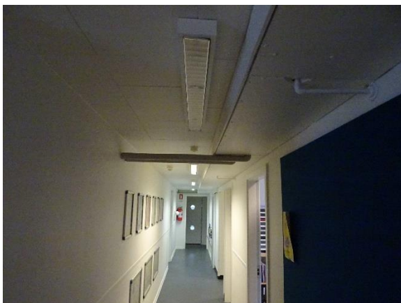
Rørkasse under loft i gang
