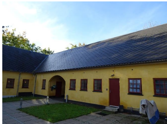
Nyeste diagonallagte eternitskifer
