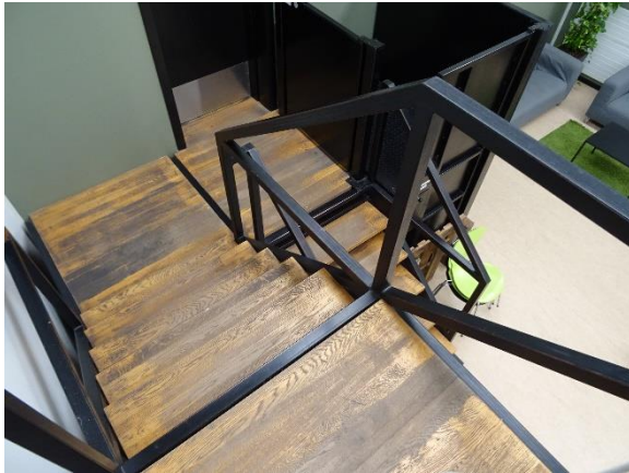
Trappe i PLC
