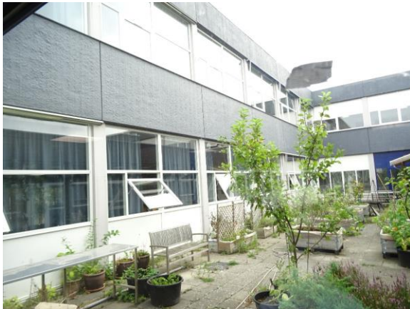
Facade mod gartneriet i gård
