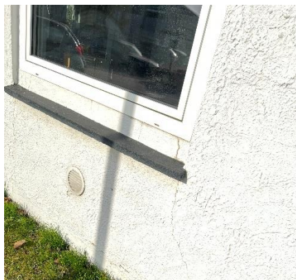
facadeisoleringen 100mm
