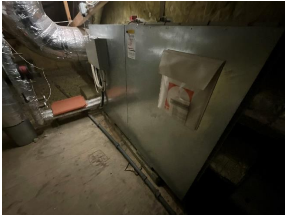
Ventilationsaggregat
