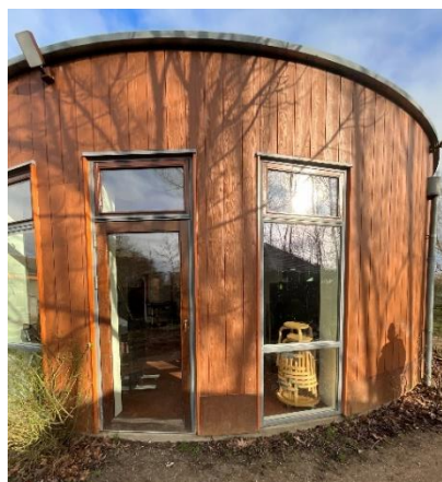
Insturation- Anex placeret bag indhegning, facade beklædt fiber cement
