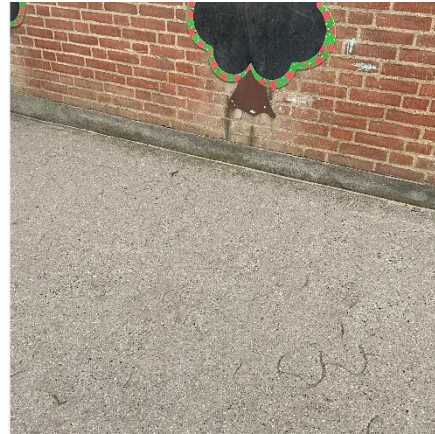
Sokkel under murfacade
