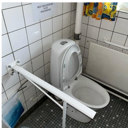
B4 To-skyls toilet
