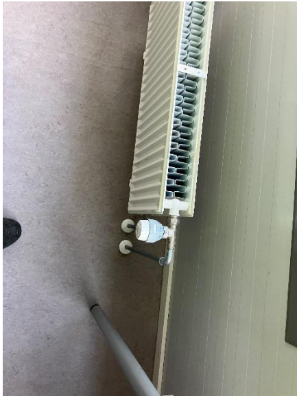
Nyere termostatventiler
