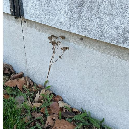
Sokkel i fibercement
