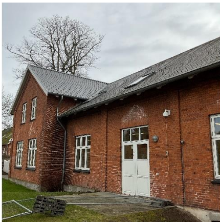
Facade mod have
