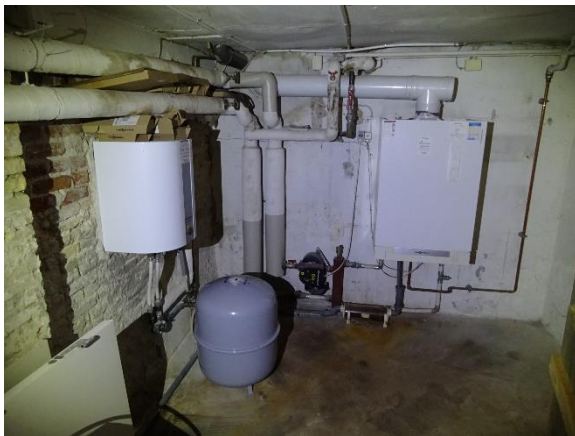
Gasfyrinstallation
