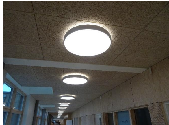
LED armaturer i gang
