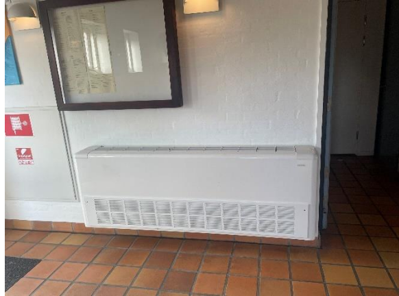
Varmpumpe inder installation i bygn.20
